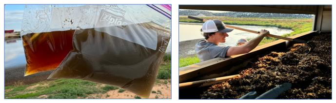
water, not adding additional nitrogen and phosphorus to irrigation fields. Now that the systems have been finetuned, it appears that the systems are doing just what was expected: removing somewhere between 85-95% of the nutrients and concentrating these nutrients in the worm beds.
